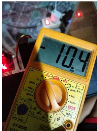
Figure 11: Motor Voltage Measurement When the Sluice Gate is Open
