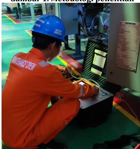
Gambar 2. Proses pengujian gas SF 6
