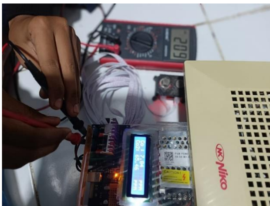
Gambar 4. Hasil pengukuran tegangan power supply
